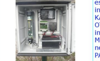
THASOS ISLAND Typical Installation of a Thalimedes™ System
